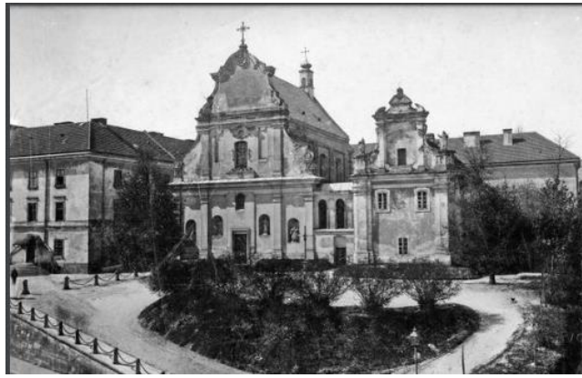
Fig. 2. Church of St. Nicholas and the old university building (Source: https://uma.lvivcenter.org/uk/photos/1707 )
