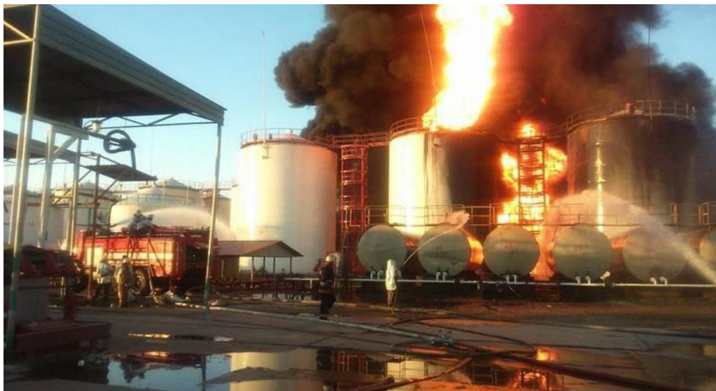
Fig. 3. Oil storage tanks explosions.
